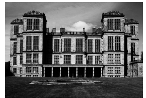
Hardwick Hall, 1590-1597 Derbyshire, UK
