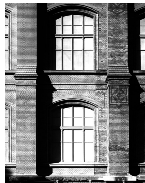
New East wing expansion at Museum of Natural History in Berlin, Diener&Diener
