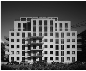
Prinsedam apartment building, Tony Fretton architects, Amsterdam, Netherlands
